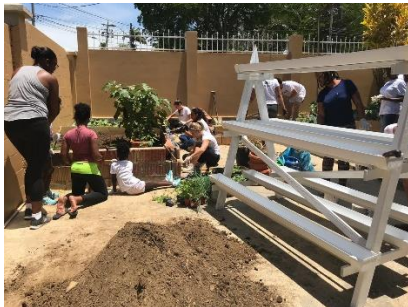
BHP installing an aquaponics feature at Rainbow Rescue
